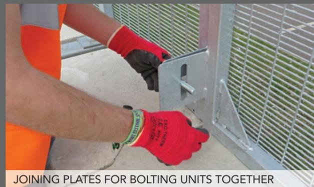
JOINING PLATES FOR BOLTING UNITS TOGETHER
