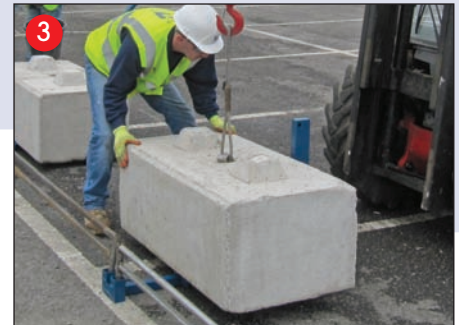
Place Ballast Block onto Base and Loading Tray (Not more than 50mm from backstop).
