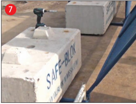
Insert Panels into Base. Manual lifting Note: Each Panel weighs 98kgs.
