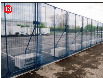
Repeat until Fence line is complete.
