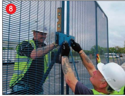
While assistants hold panels vertical, fit 4no. M8x70 Coach Bolts through Front Clamp Plate, Panel Mesh and Brace Plate using Nyloc Nuts and M8x50 Washers behind.
