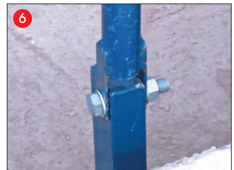
Connect Brace to Base using M16 Hex Bolt and Washers.
