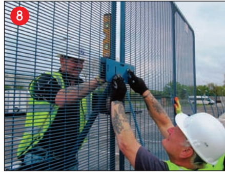
While assistants hold panels vertical, fit 4no. M8x70 Coach Bolts through Front Clamp Plate, Panel Mesh and Brace Plate using Nyloc Nuts and M8x50 Washers behind.
